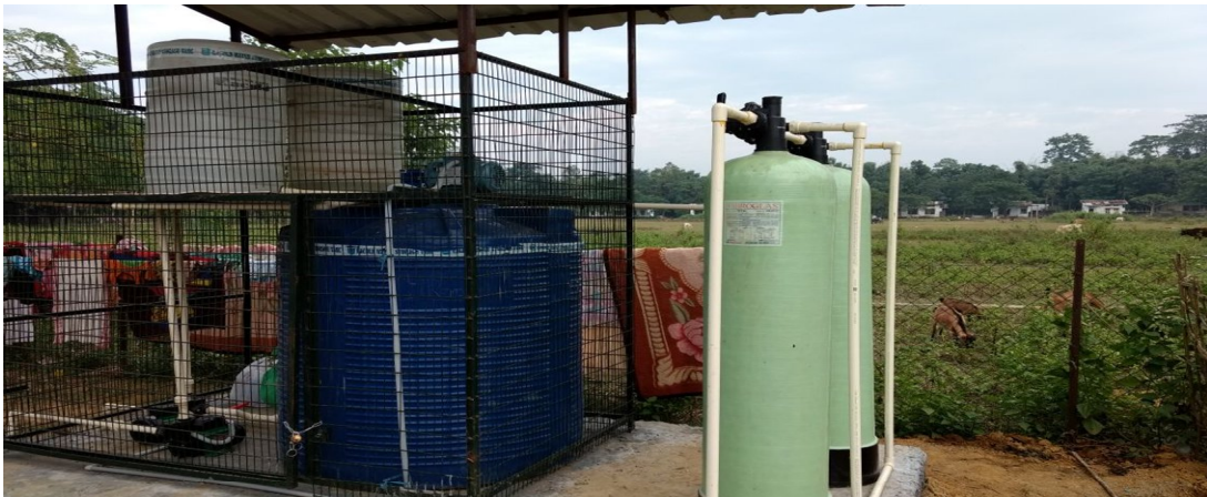
Effluent Treatment Plant for liquid infectious waste
